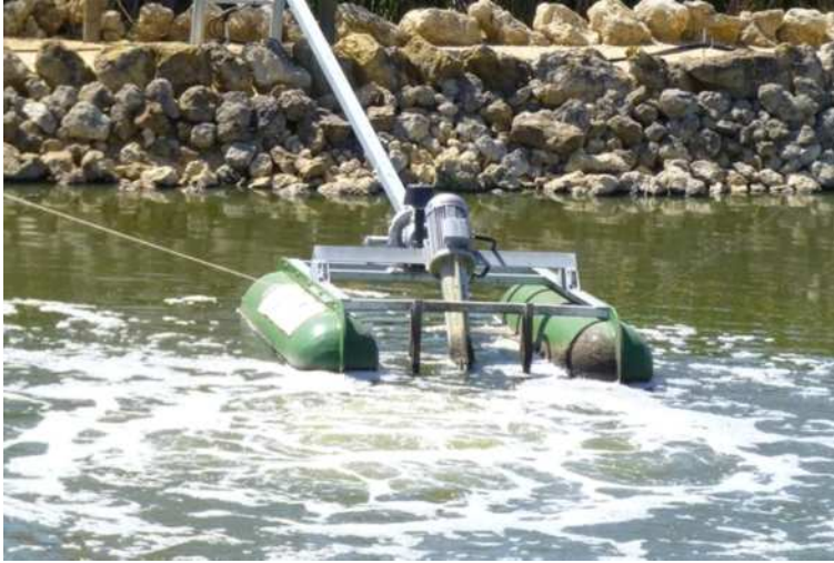
Aerated Wastewater Lagoon System in Spain (700 PE)
